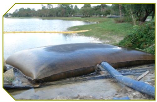
Dewatering Operations are practices that manage the discharge of pollutants when non-storm water and accumulated precipitation must be removed from a work location so that construction work may be accomplished. A Dewatering Bag / Tube, is a square or rectangular bag made of non-woven geotextile fabric that collects sand, silt, and fines.
